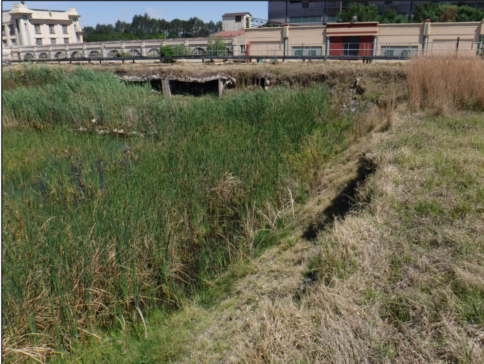
Plate 7. North-western corner of old System 1A excavation, which is partially filled with water.
