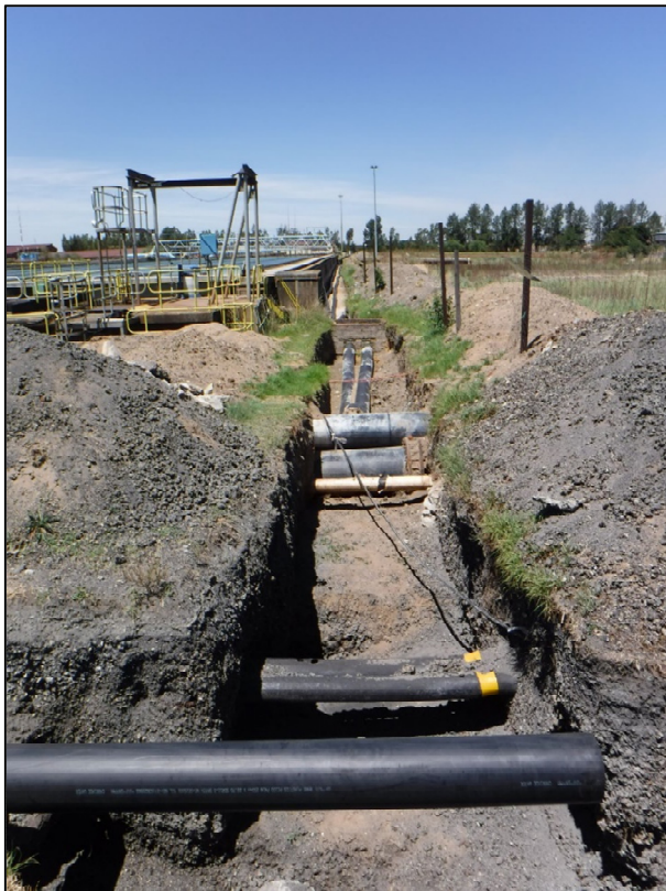
Plate 6. Large number of services visible in one of the trench excavations.
