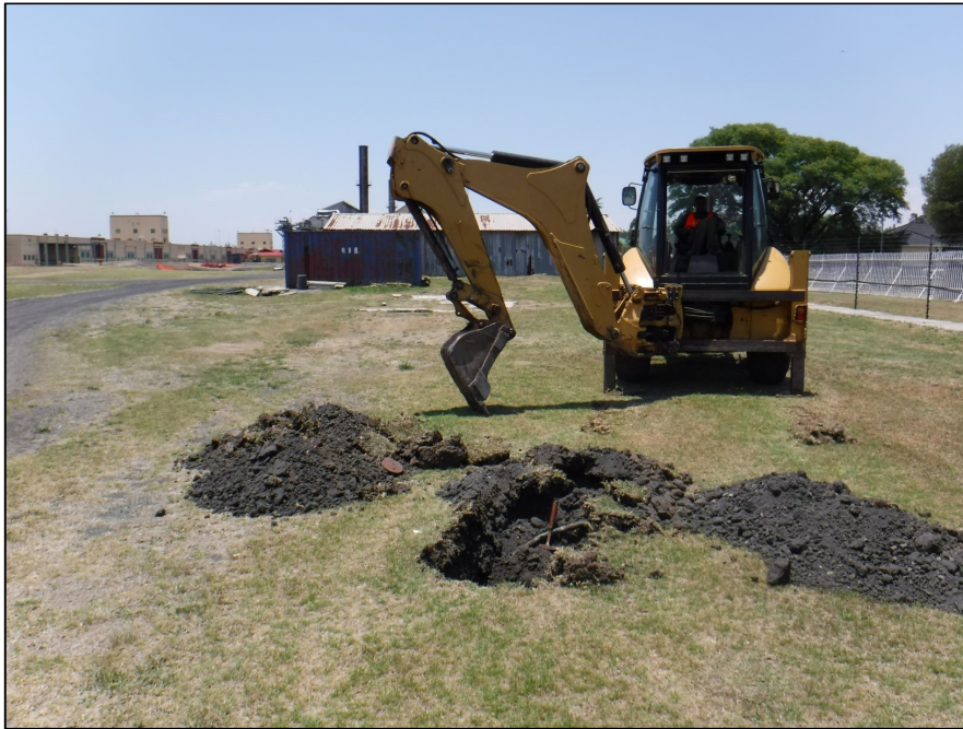
Plate 1. TP1 excavation with a TLB in progress.
